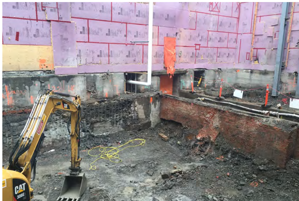
▲ Ticketing Block - Excavation of New Full Basement (JCAL 2017)
