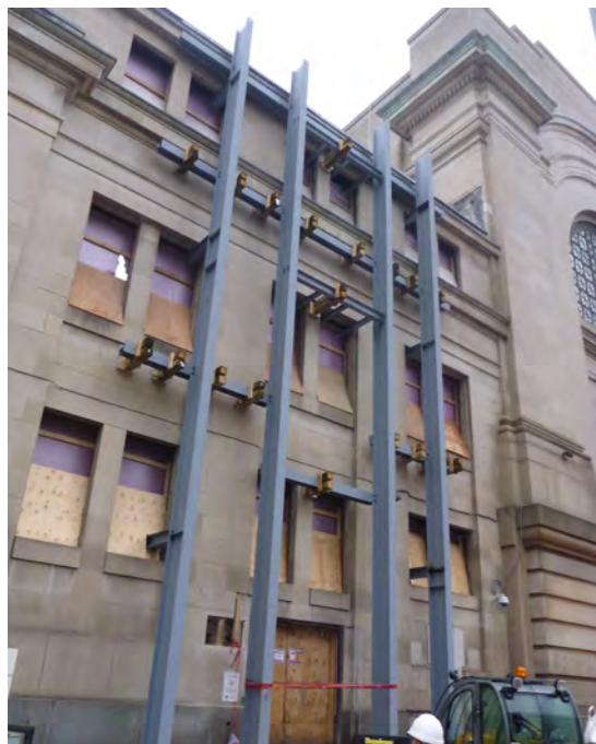
▲ Ticketing Block - Shoring Exterior Walls (JCAL 2017)
