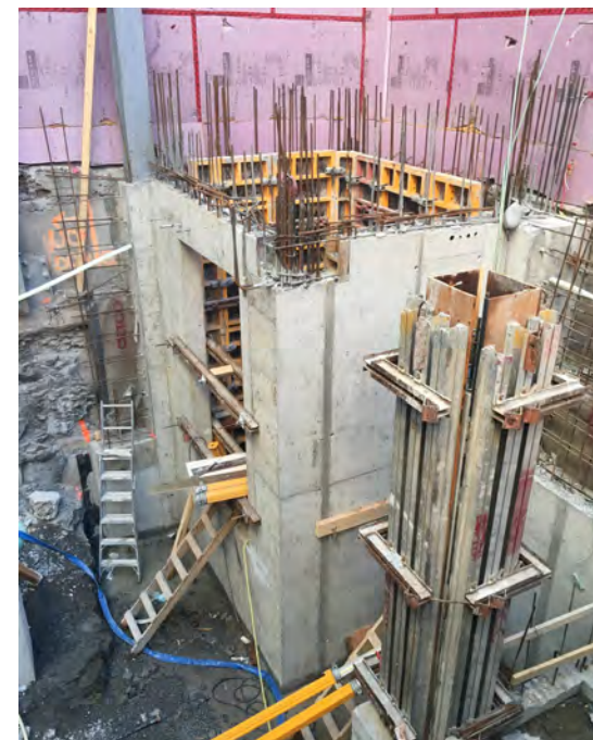
▲ Ticketing Block - New Concrete Shear Walls (JCAL 2017)
